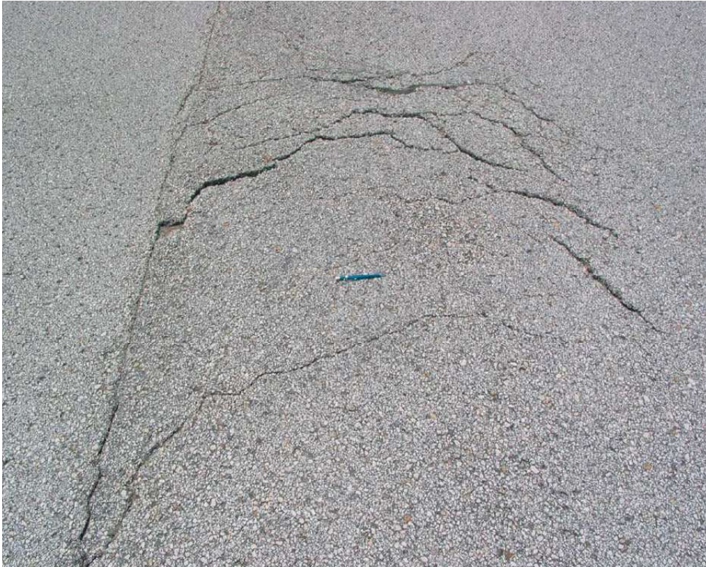
Figure C.10: Slippage Cracking.
