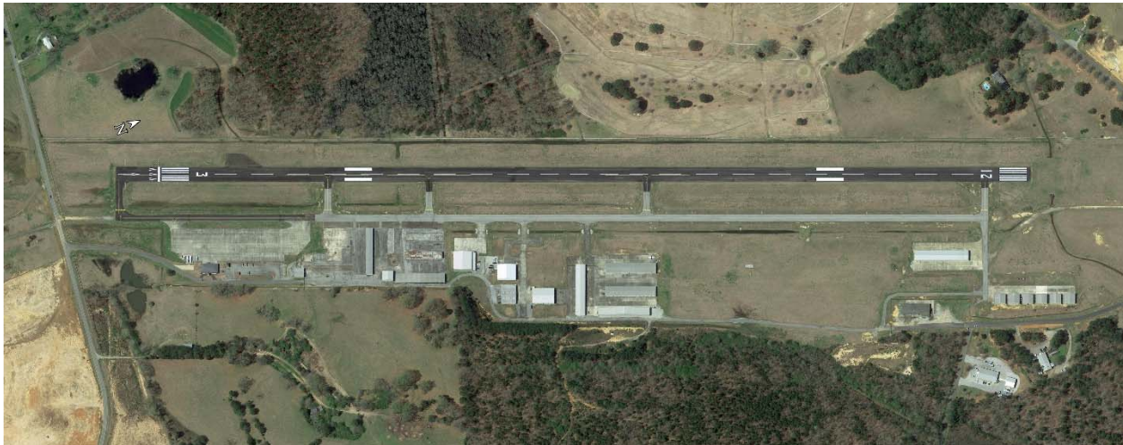
Figure 2.1: St Clair County Airport.
