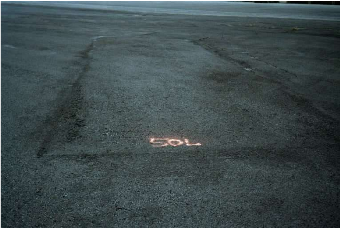
Figure C.7: Asphalt Patching.
