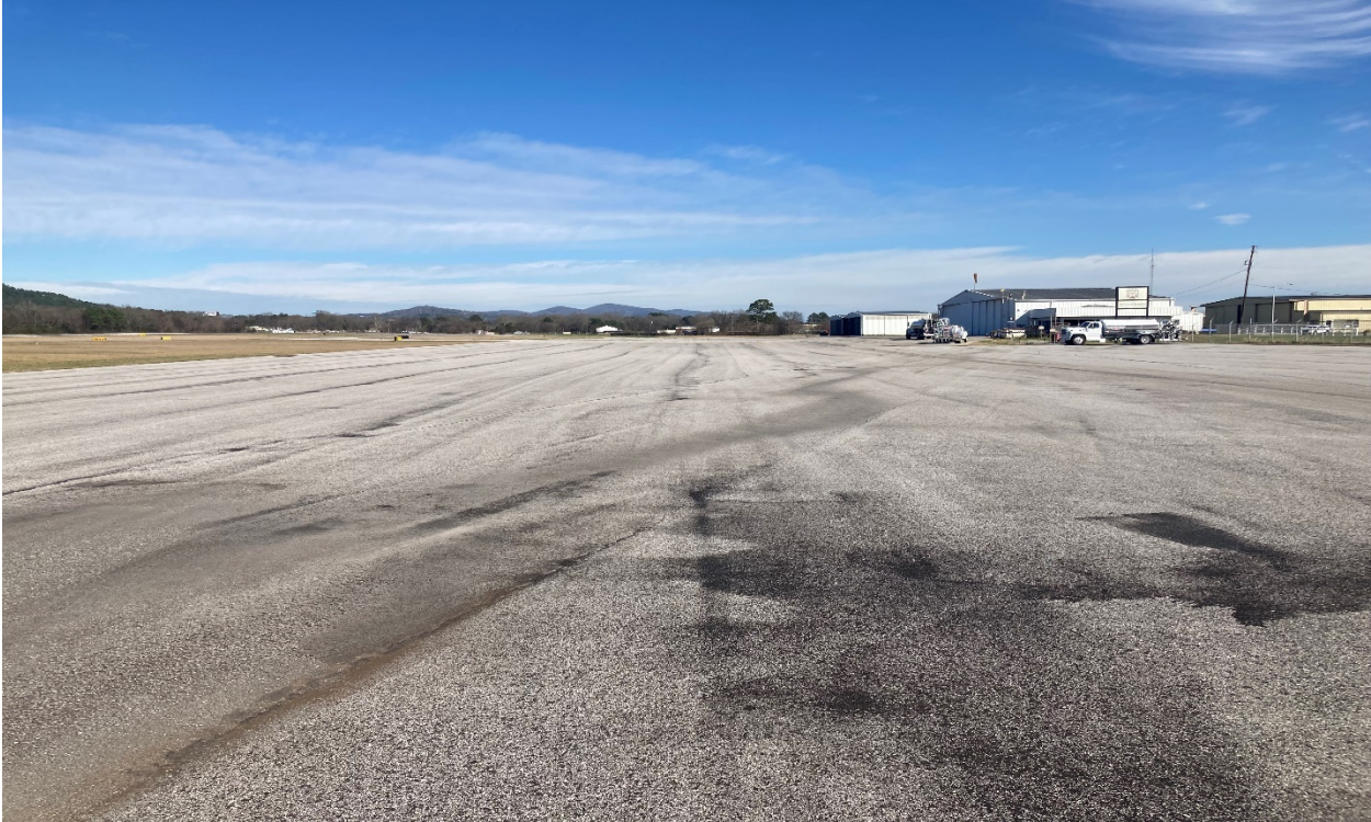
Photo #9 – Main Apron
