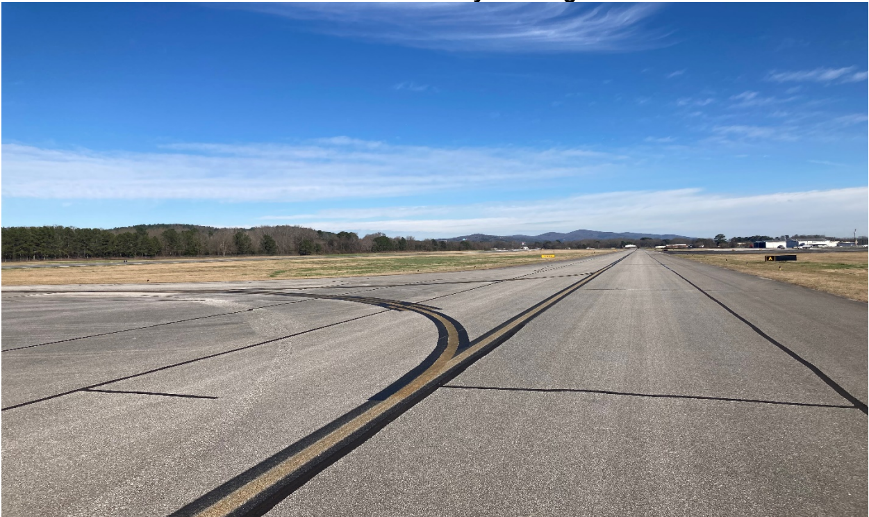
Photo #5 – Taxiway Markings
