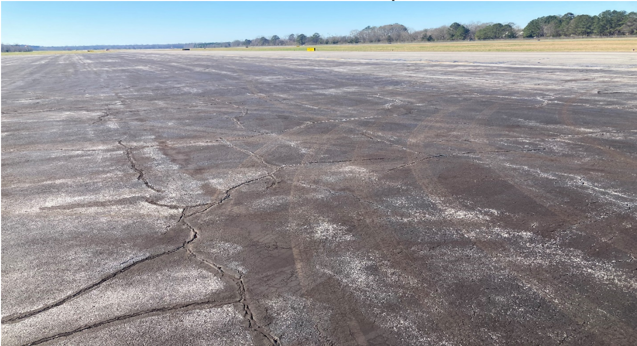
Photo #10 – Terminal Apron
