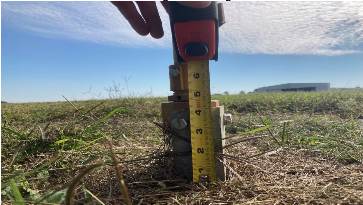
Photo #3 – Light Fixture Angle Iron
