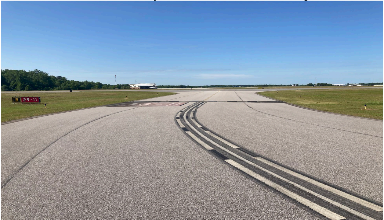
Photo #7 – Taxiway B Enhanced Centerline Markings
