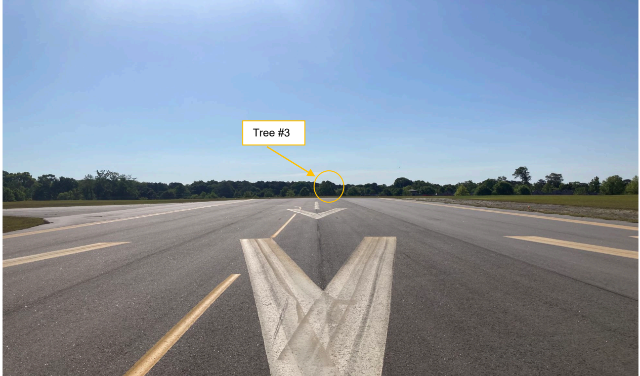
Photo #3—Runway 29 Approach
