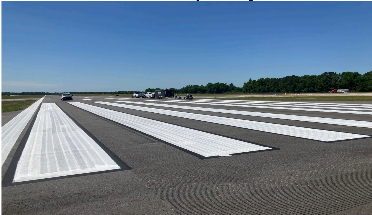
Photo #5 – Runway 18 Markings
