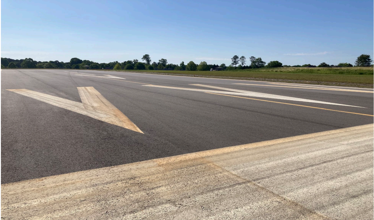
Photo #6 – Runway 29 Markings
