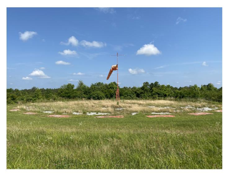
Wind direction indicator is in <u>FAIR</u> condition. However, the paint on the segmented circle is beginning to fade and chip. <u>Maintenance:</u> Repaint the segmented circle.
