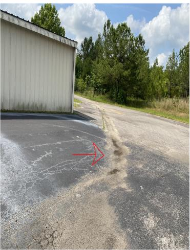
The taxiway surface is generally in **GOOD** condition. However, there is one portion of the taxiway surface that leads to hangars that is in **POOR** condition. Additionally, the surface around the hangars has a substantial amount of FOD on the pavement surface.
