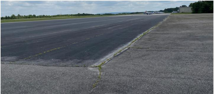
The main apron surface in front of the terminal building is in **FAIR** condition. However, the apron located Southwest of the terminal apron is in **POOR** condition. Additionally, the Apron surface is in poor condition and experiencing moderate cracking and vegetation growth.
