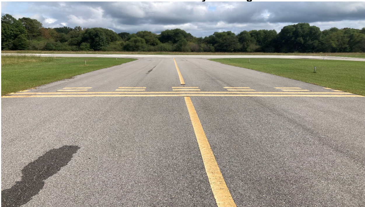
Photo #5 – Taxiway Markings
