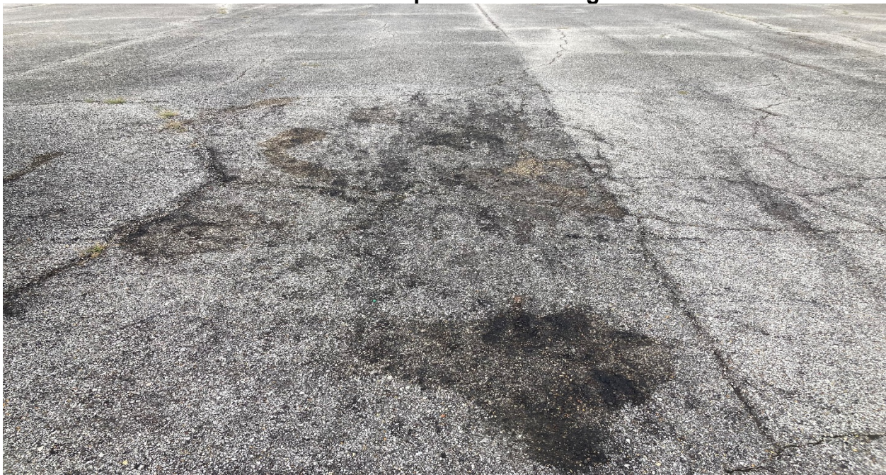
Photo #8 – Apron Skid Damage
