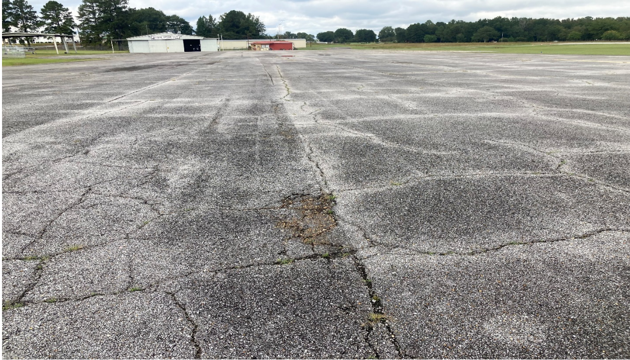
Photo #8 – Apron Skid Damage
