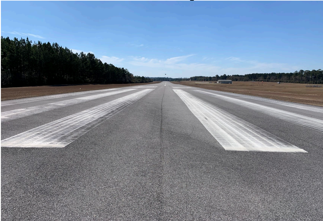
Photo # 5 – NPI Markings RWY 22
