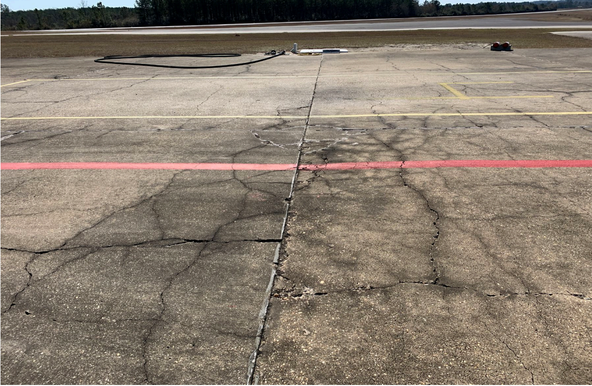
Photo # 10 – Hot Refueling Apron
