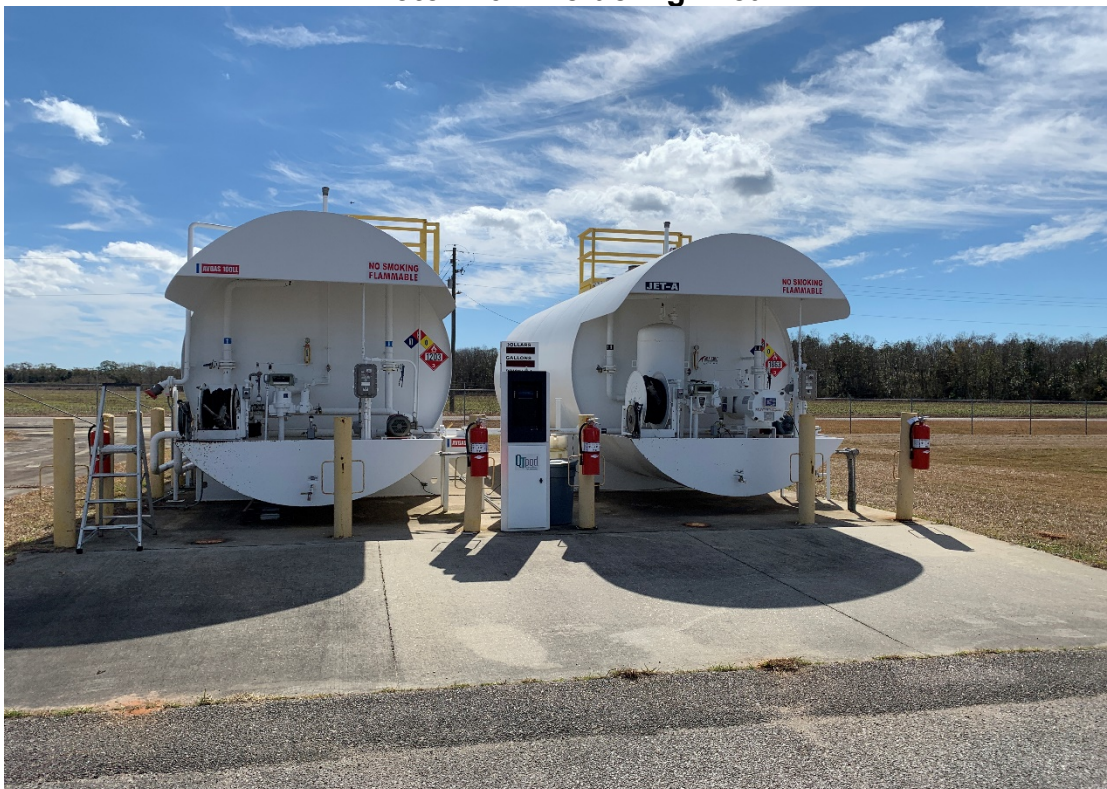
Photo #10 – Refueling Area
