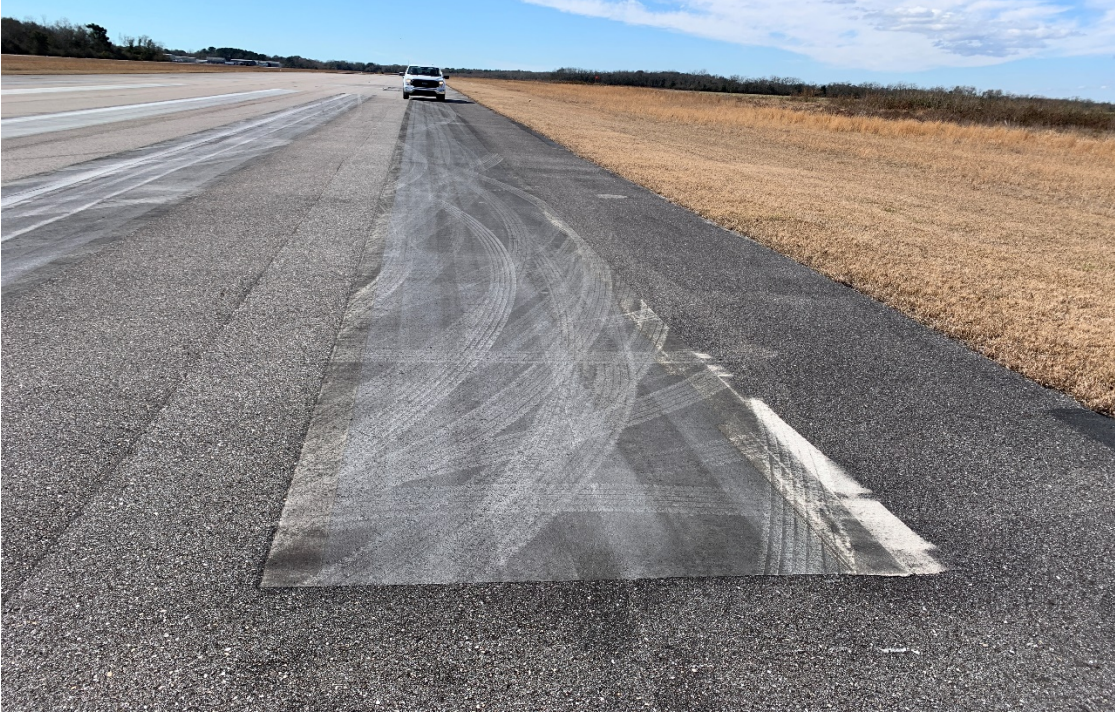
Photo # 5 – NPI Markings Runway 24
