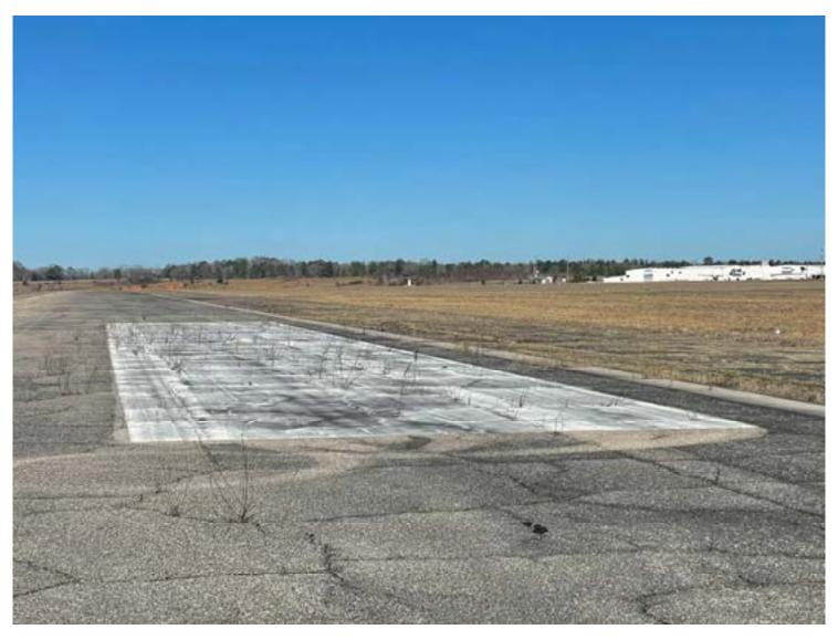
Runway markings are in **<u>POOR</u>** condition. Maintenance: Runway should be cleaned of all vegetation.
