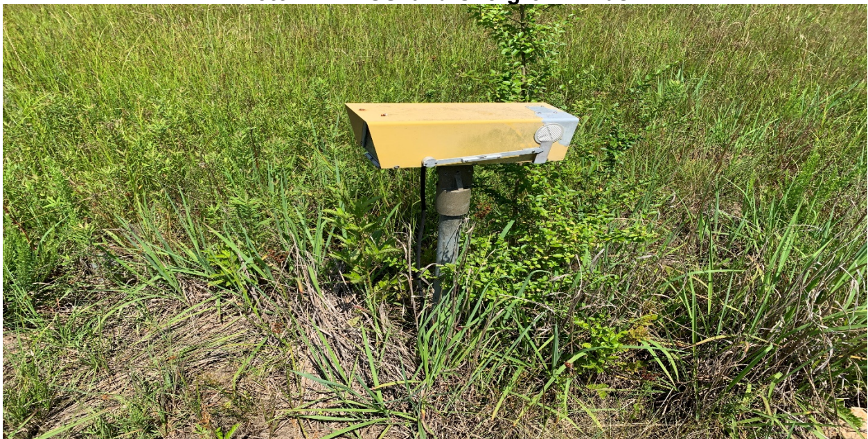
Photo # 4 – VGSI and Overgrown Brush
