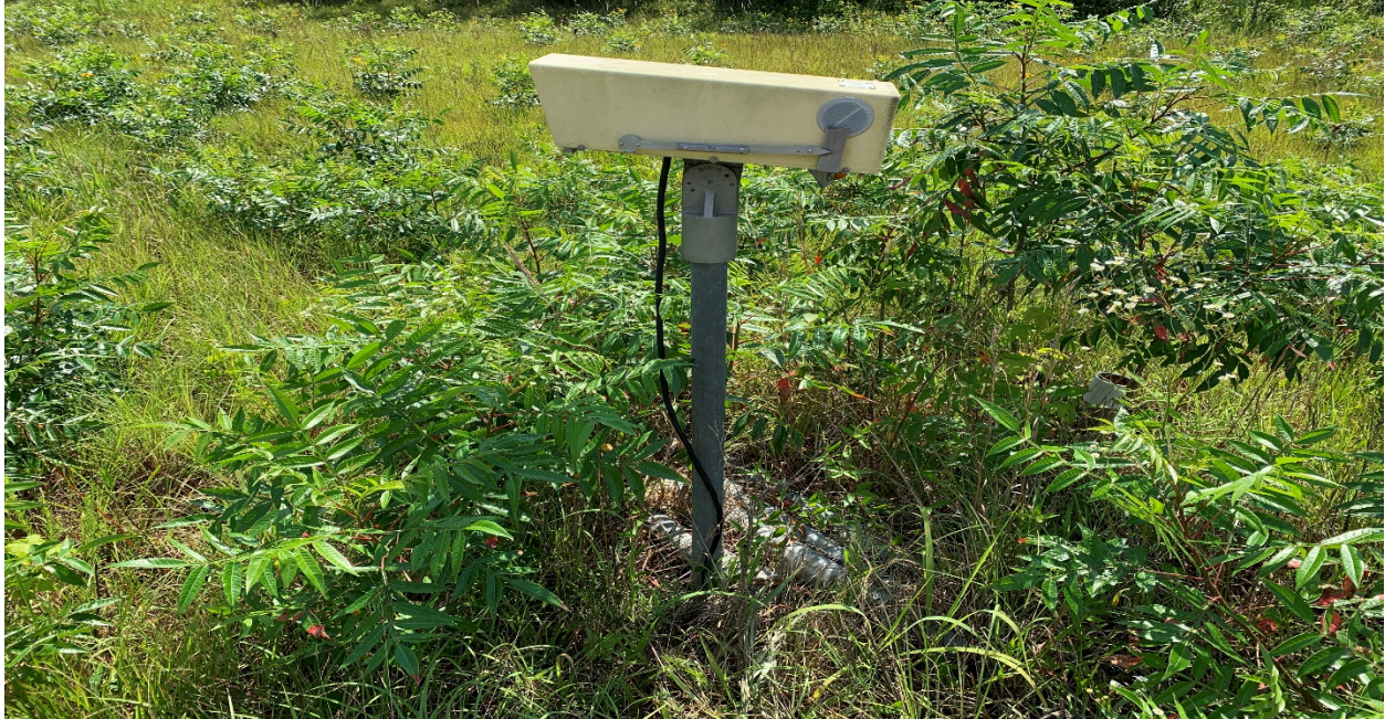
Photo # 3 – VGSI and Overgrown Brush
