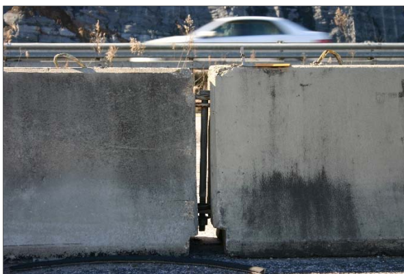
✓ Good Condition (Bolt and Loop Type)
