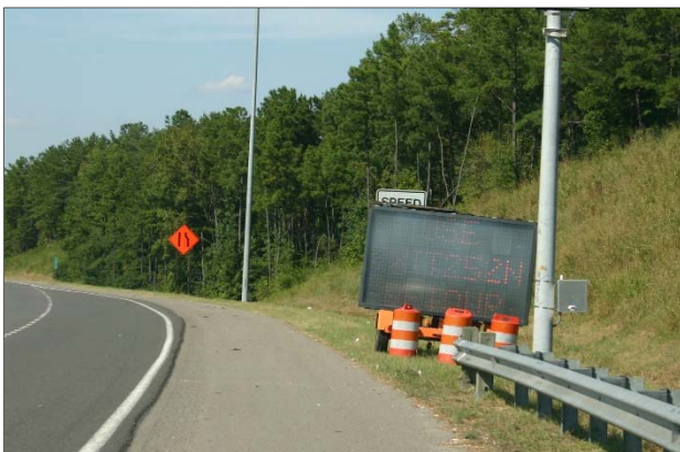
X Too Low, Not Levelled, Blocking Other Sign
