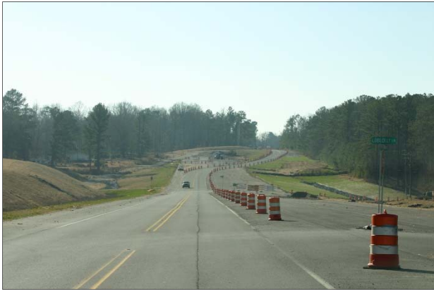
✓ Good Spacing and Alignment
