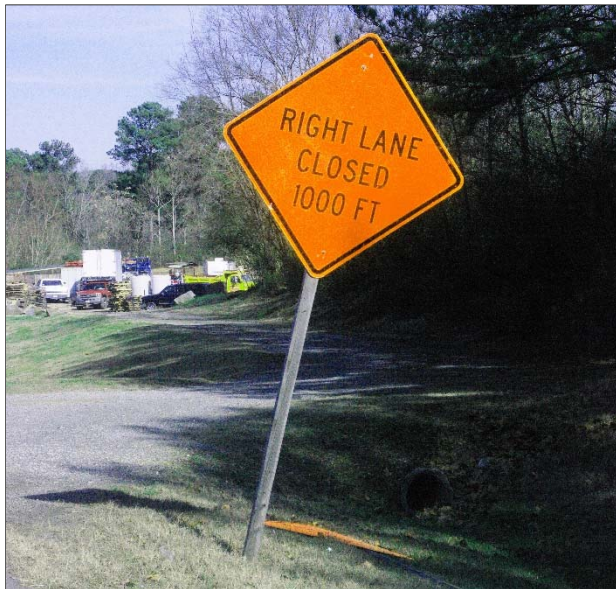
X Out of Plumb
