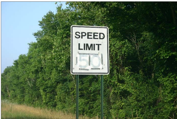
X Improper Sign Cover
