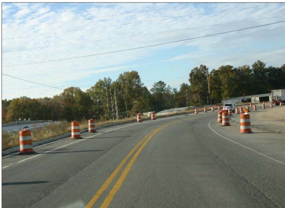
X Poor Spacing
