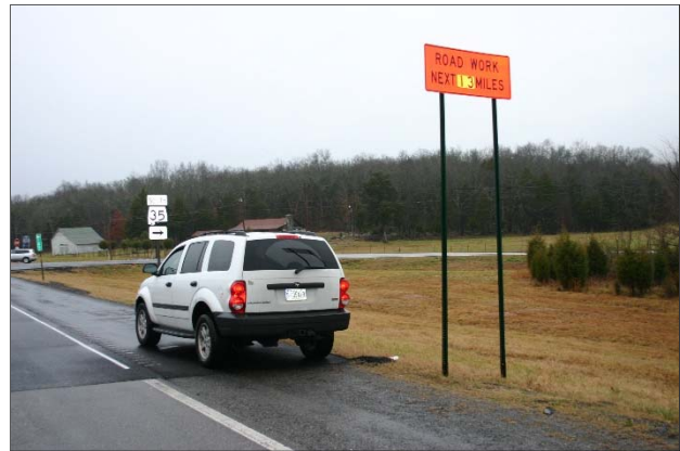
X Excessively High Mounting
