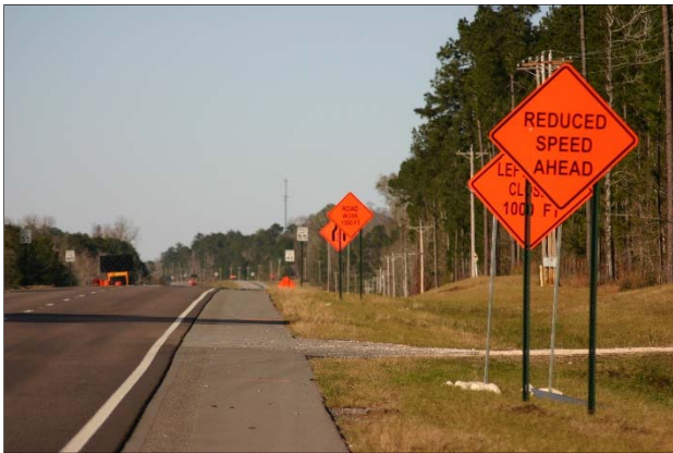
X Inadequate Space Between Signs
