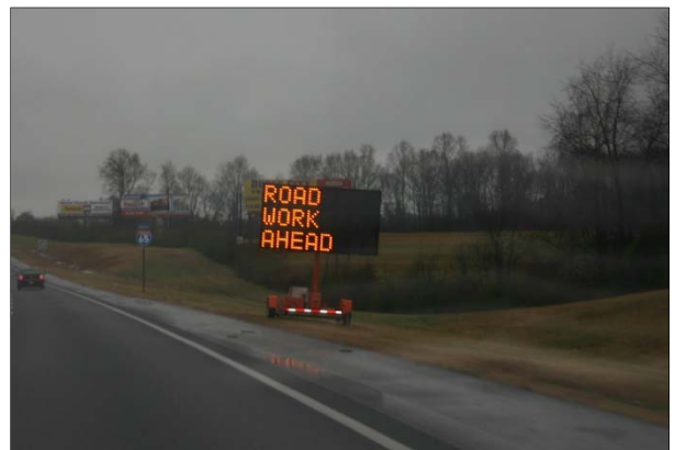
X Not Delineated with Drums
