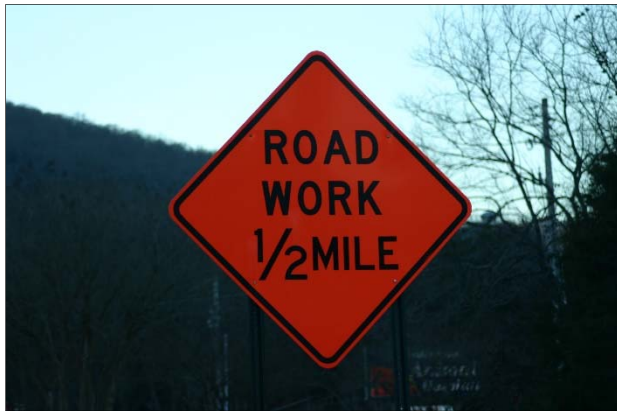
✓ Good Condition and Visibility
