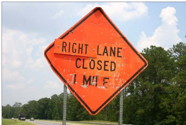
X Scratched and Damaged Sheeting
