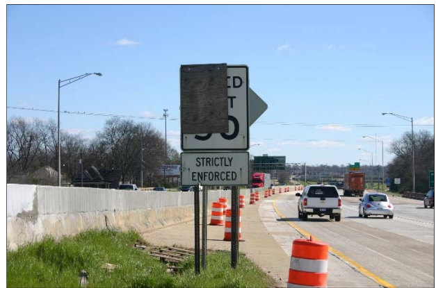
X Improper Sign Cover
