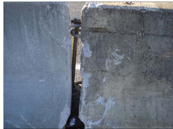
X Not Bolted at Bottom
