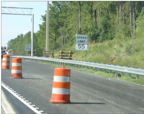
X Conflicting Speed Limit Signs
