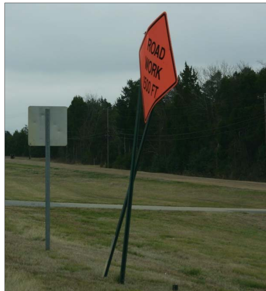
X Damaged Posts
