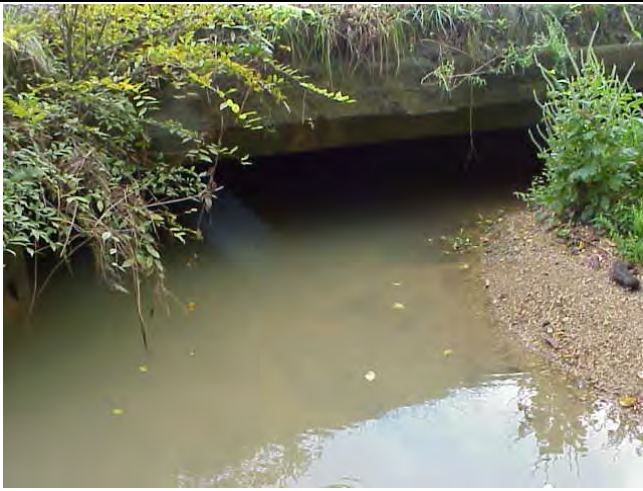
Site 1 (Stream 1) facing downstream.
