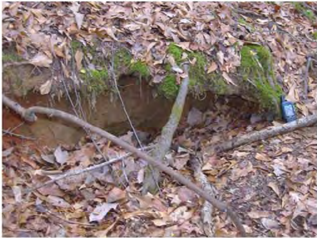
Roof collapse area in the northern part of the study area along Alternate I
