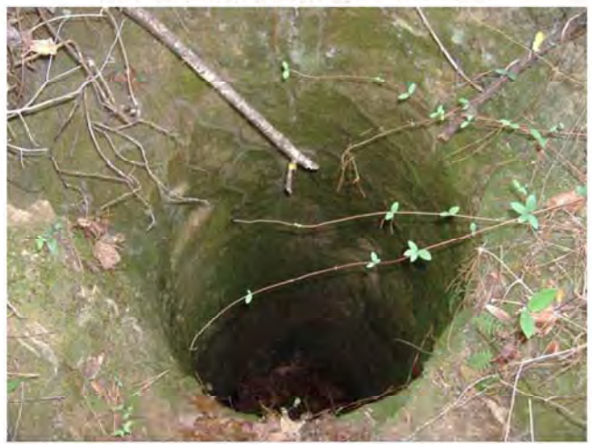
Air shaft in the southern part of the study area to the southeast of Alternate I
