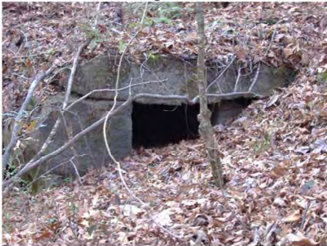
Old Railroad culvert in central part of the study area
