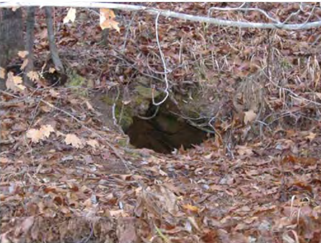
Roof collapse area in the central part of the study area along Alternate II
