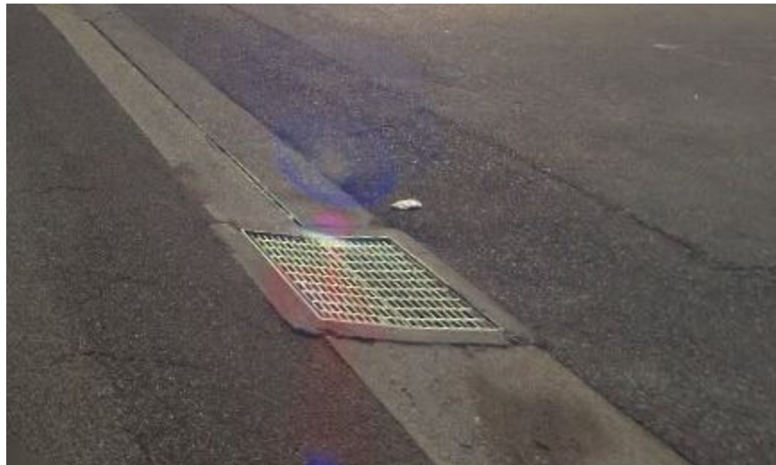
Figure 6.4 - Photograph of typical V-inlet
