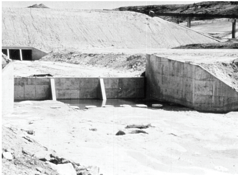
Figure 8.23 – Straight drop spillway stilling basin
