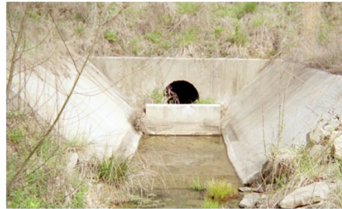
Figure 8.27 (left) – Schematic of Contra Costa Energy Dissipator
