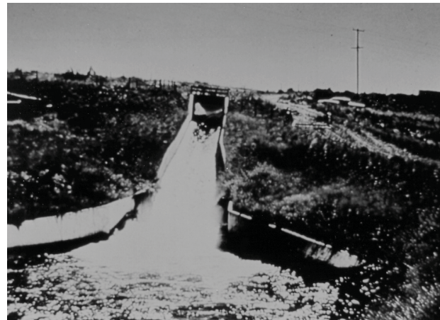
Figure 8.19 (left) – Schematic of SAF stilling basin
