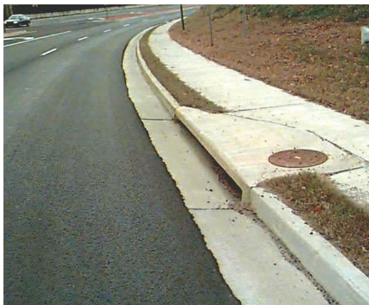
Figure 6.7 - Curb inlet placed on continuous roadway grade
