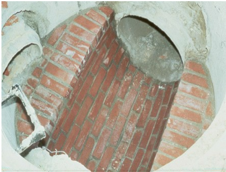
Figure 7.10 - Example of a bench in an access hole
