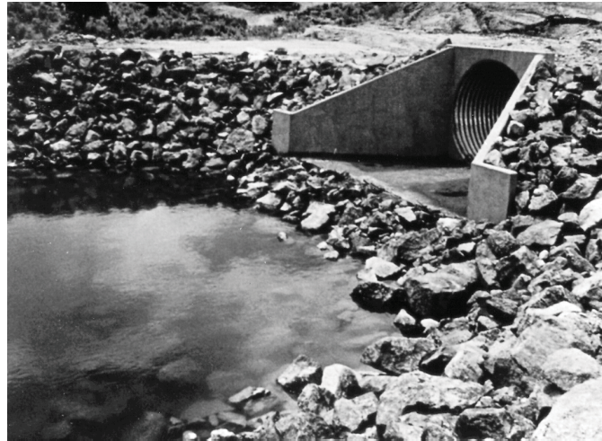
Figure 8.26 – Riprapped culvert energy basin
