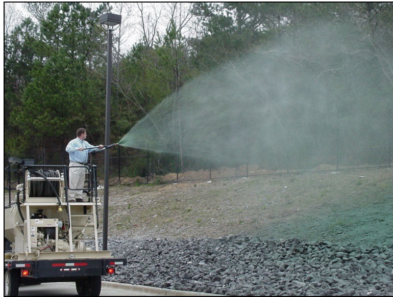
Photo courtesy of Sunshine Supplies, Inc.
