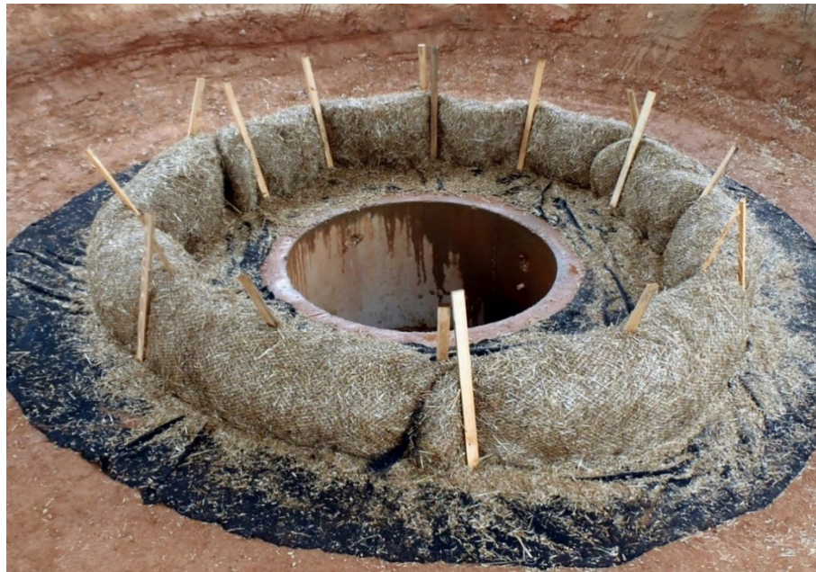
Figure IP-6 Wattle Inlet Protection Installation.
