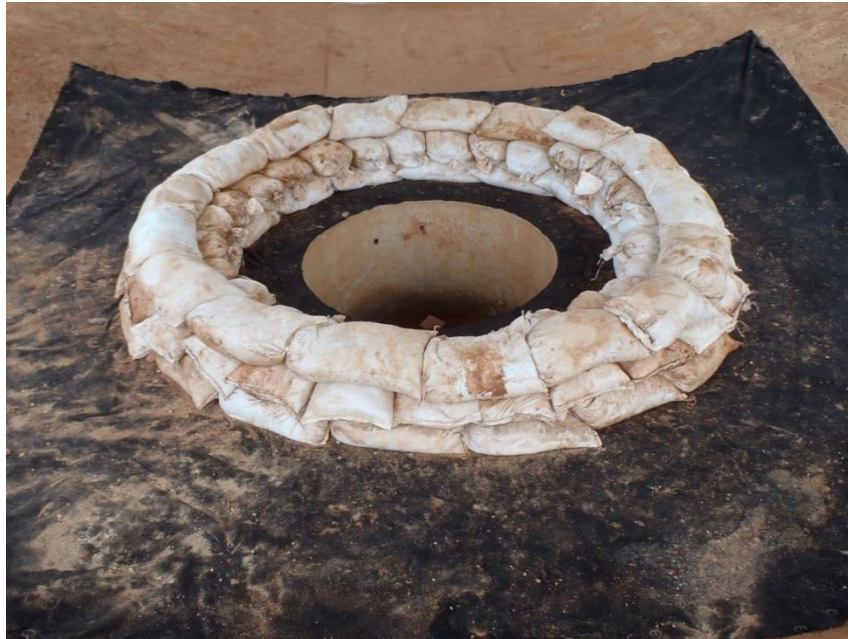
Figure IP-4 Sand Bag Inlet Protection Installation.
