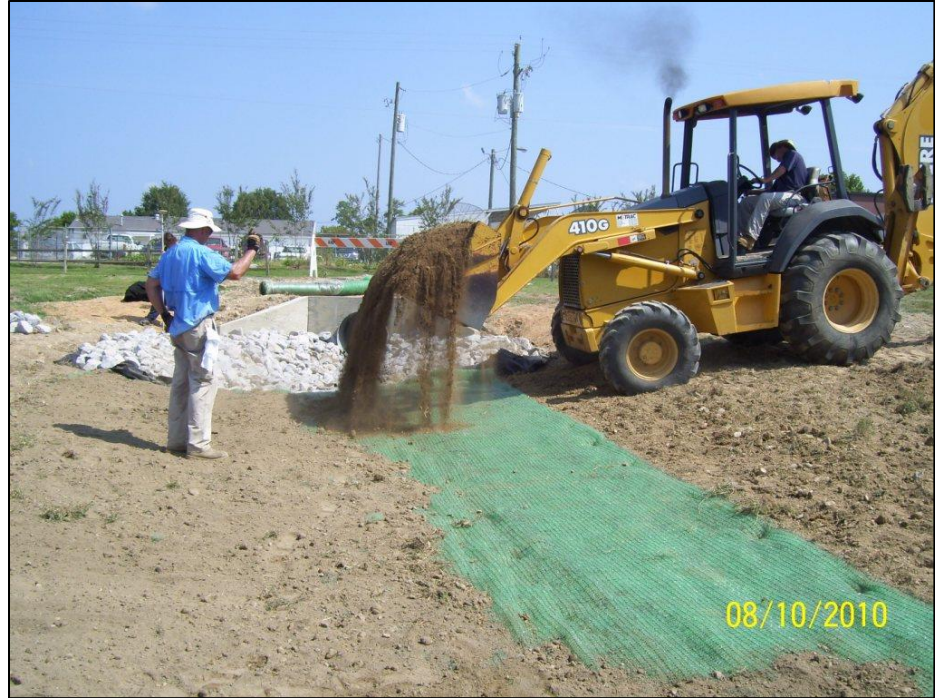
Figure ECB-2 Topsoil "In-Fill" Being Placed in TRM.
