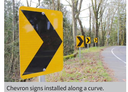
Chevron signs installed along a curve.
