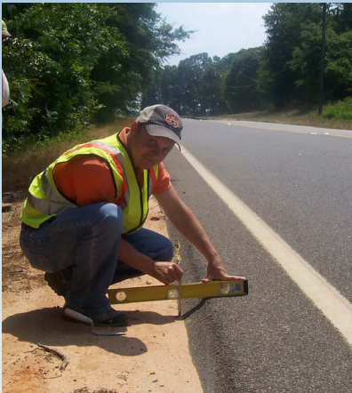
Example of SafetyEdge SM after backfill material settles or erodes.
