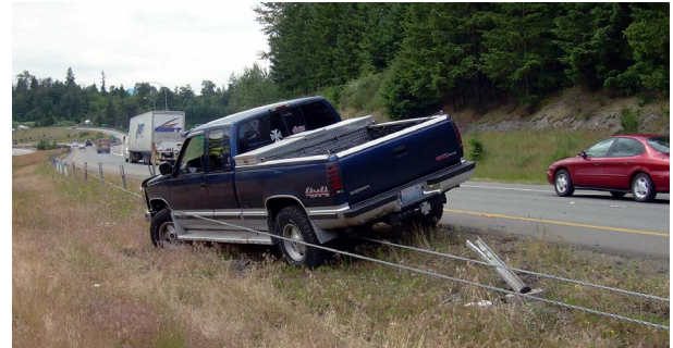
Median cable barrier prevents a potential head-on crash.
