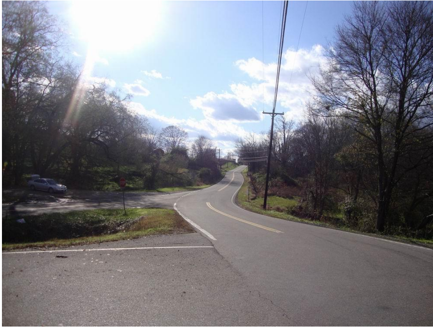
Photo 7: Looking southwest along SR-33 at the intersection with SR-22
