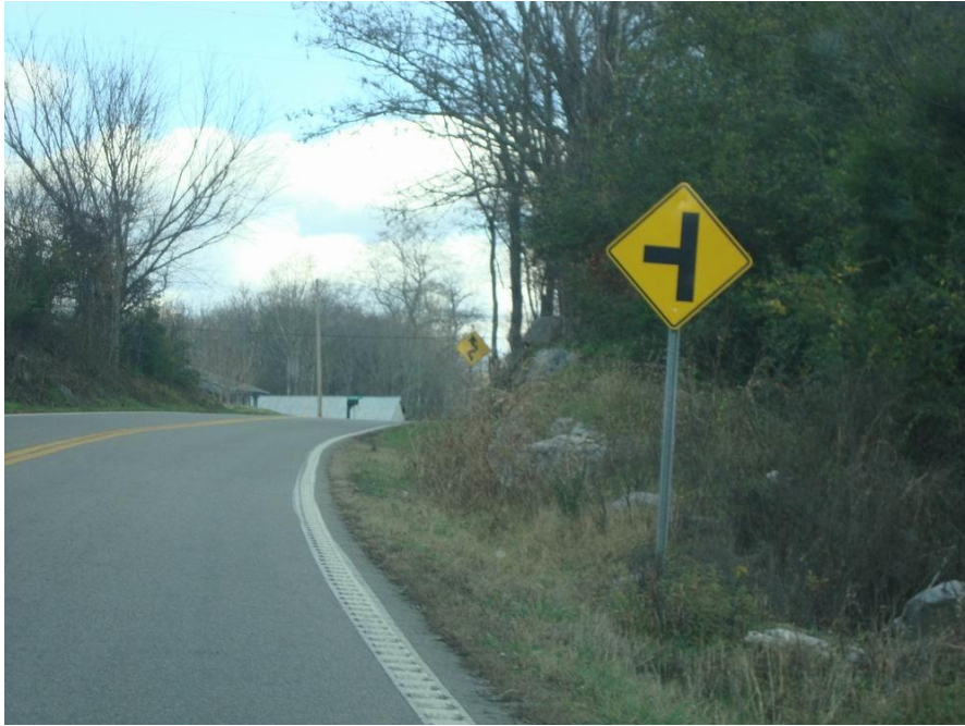
Photo 9: Looking northeast along SR-22 approaching Creek Road
