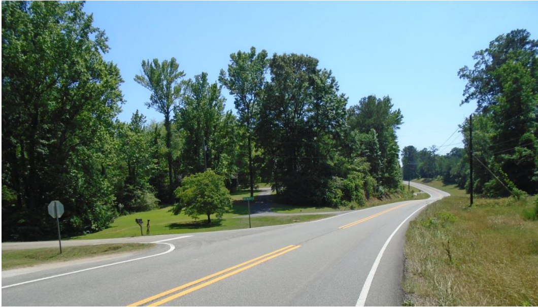
CR-216 looking east at mile point 26.1
