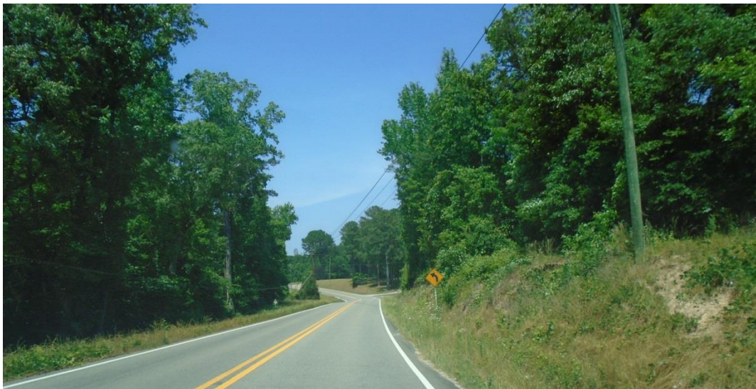
CR-216 looking west at mile point 26.2
