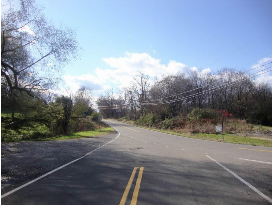
Photo 3: Looking southwest along SR-33 at the SR-22 intersection
