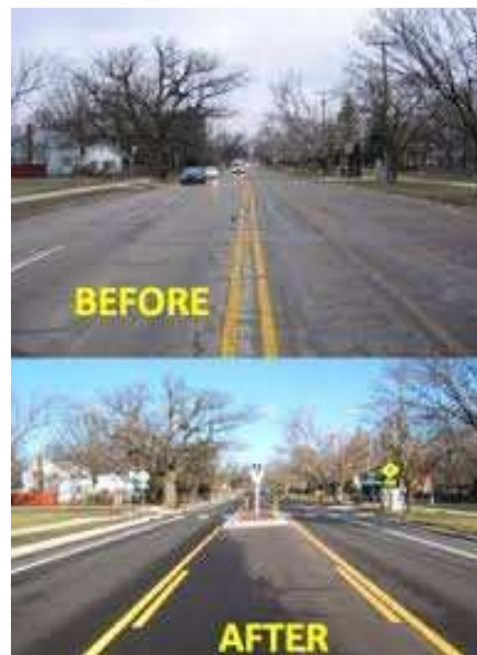
Figure 23. Example of “Before” and “After” of a Road Diet
