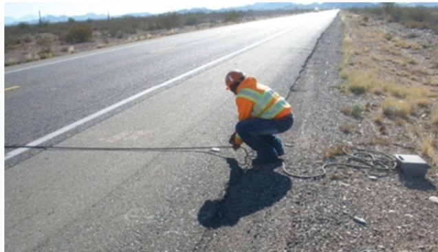
Figure 1. Pneumatic Road Tube Counter Installation
