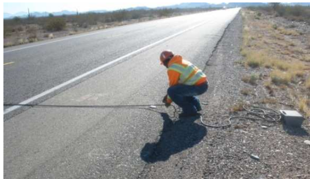
Figure 5. Pneumatic Tube Counter Example
