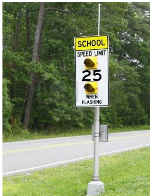
Figure 14. Flashing School Speed Limit Sign
