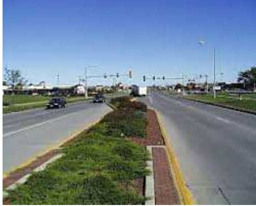
Figure 24. Raised Median Example
