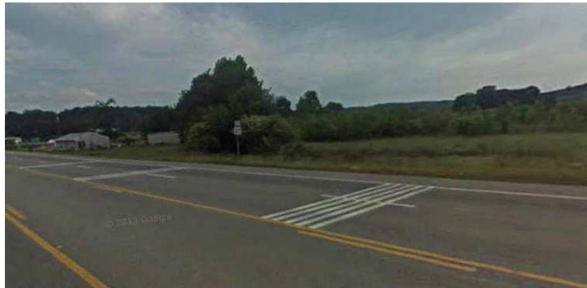
Figure 19. Transverse Rumble Strips
