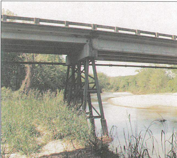
Combination Concrete Spans
