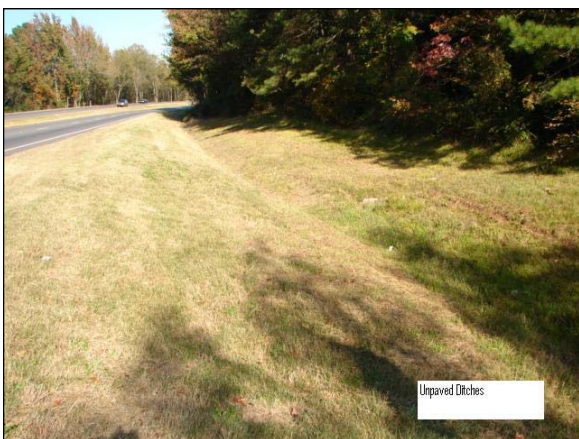
Functional Unpaved Ditch Condition - Do Not Count as Deficient
