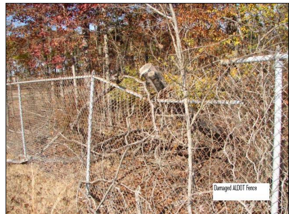
Deficient ALDOT Fence – Count Linear Feet of Deficiency
