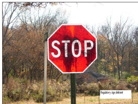
Deficient “Regulatory Sign” Sample – Count as Deficient
