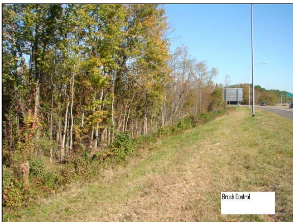
Functional Brush/Tree Control Condition - Do Not Count as Deficient
