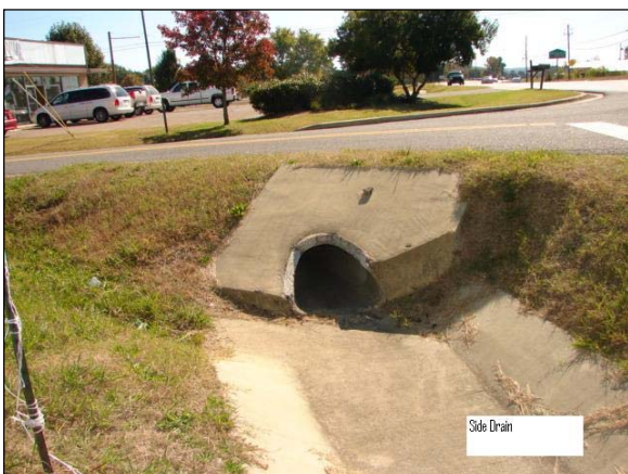
Functional Side Drain Condition - Do Not Count as Deficient
