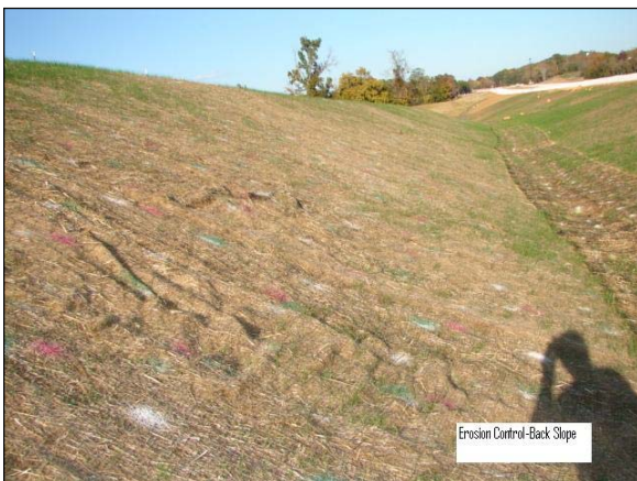
Functional Back Slope Condition - Do Not Count as Deficient
