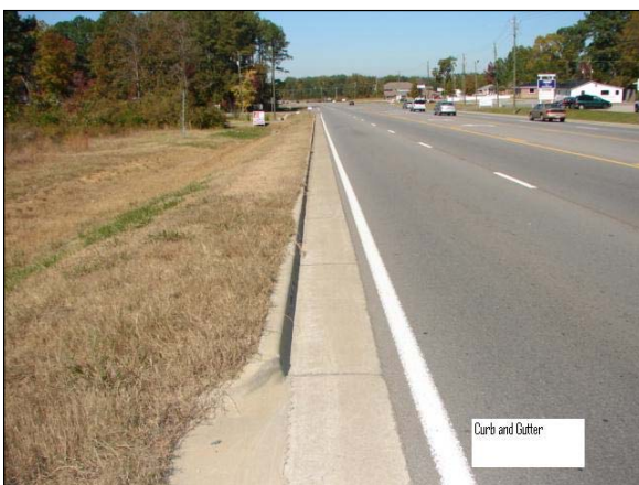
Functional Curb and Gutter Condition - Do Not Count as Deficient
