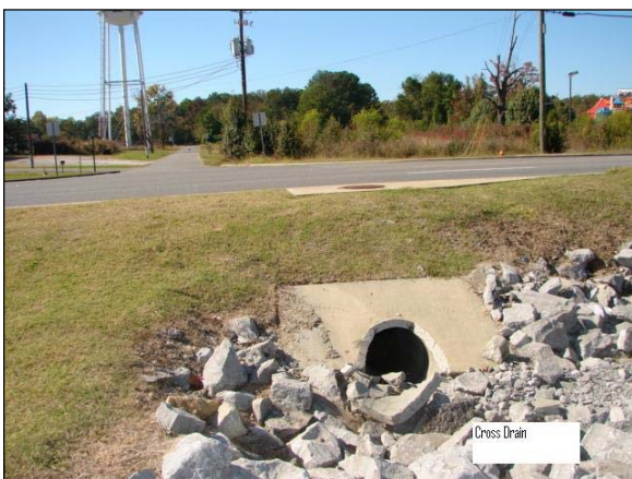
Functional Cross Drain Condition - Do Not Count as Deficient
