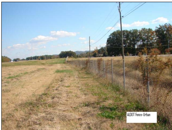
Functional ALDOT Fence – Do Not Count as Deficient
