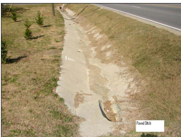
Functional Paved Ditch Condition - Do Not Count as Deficient
