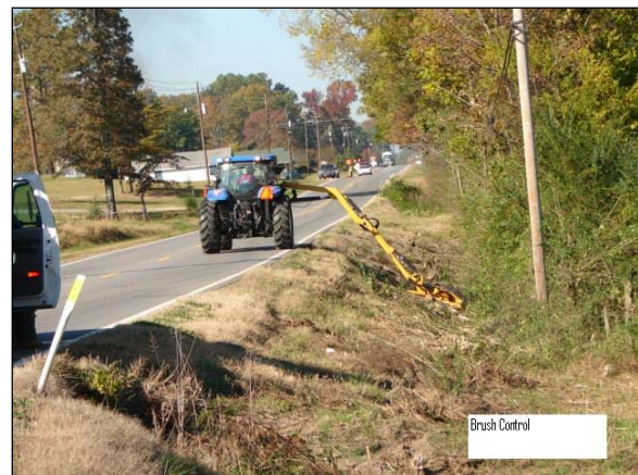
Deficient Brush/Tree Control Condition - Count Linear Feet of Deficiency
