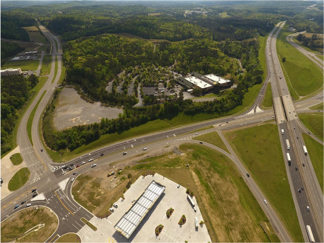
Figure E-28: After Interchange Improvements
