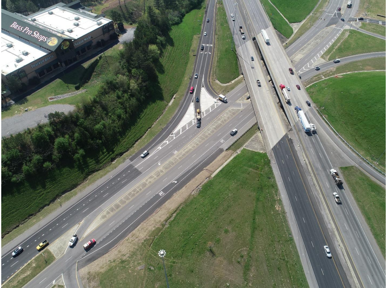
Figure E-29: After Interchange Improvements
