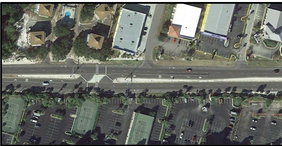
Figure 2-8: Alabama Highway 182 in Orange Beach, Alabama After Access Management
