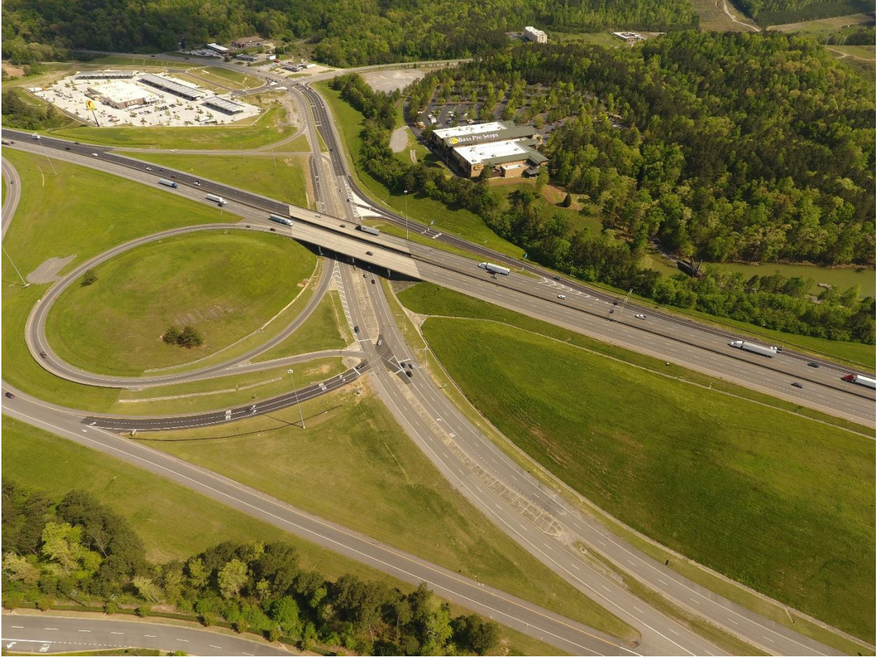
Figure E-27: After Interchange Improvements
