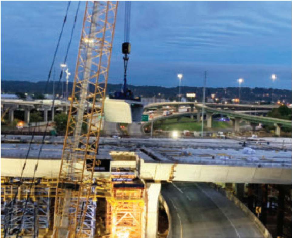
A view of a segment being placed onto the I-59/20 bridge
