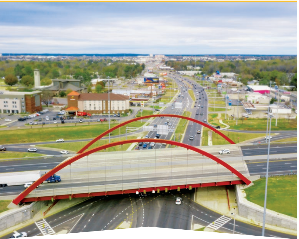
The crimson arched bridge on I-20/59 over McFarland Avenue welcomes drivers headed into Tuscaloosa.
