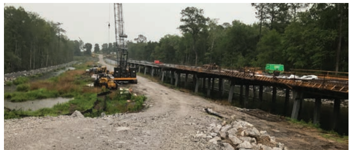
ALDOT is extending the eastbound bridge over Big Creek.
