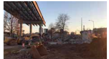
Demo of CBD Bridges over Carraway Boulevard.
