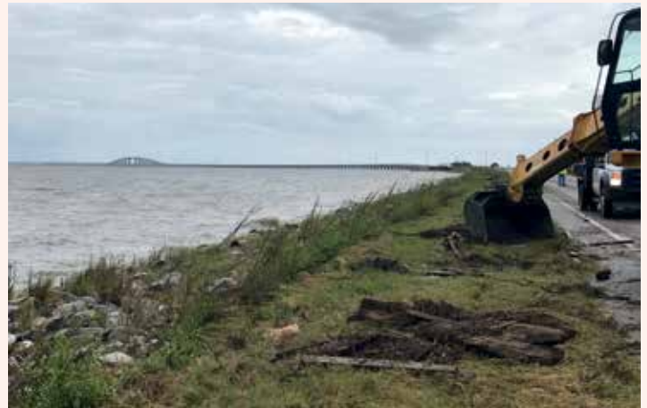
Debris being removed on Dauphin Island Parkway.
