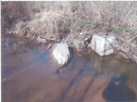
(28) Erosion around J-hook 7 has caused the rocks to fall into channel.
