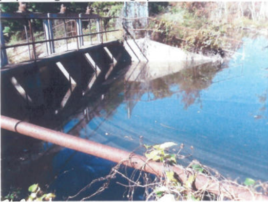
(42) Floodgate is backing up excessive amount of water in natural wetlands.
