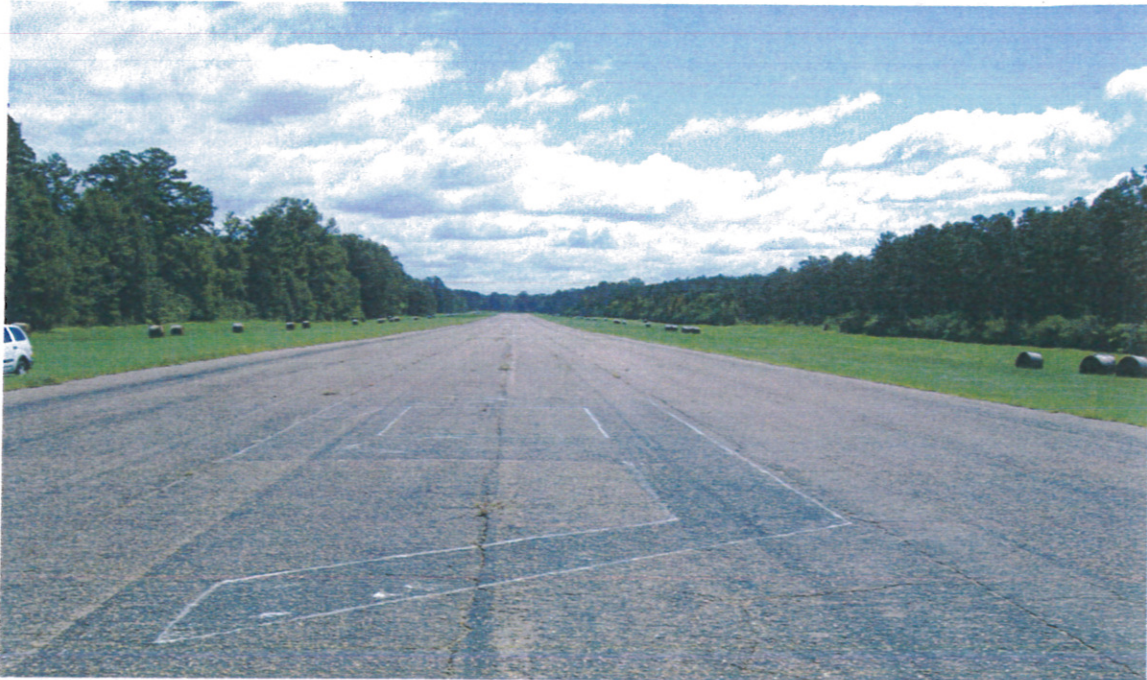
Photo # 4 – Runway Markings
