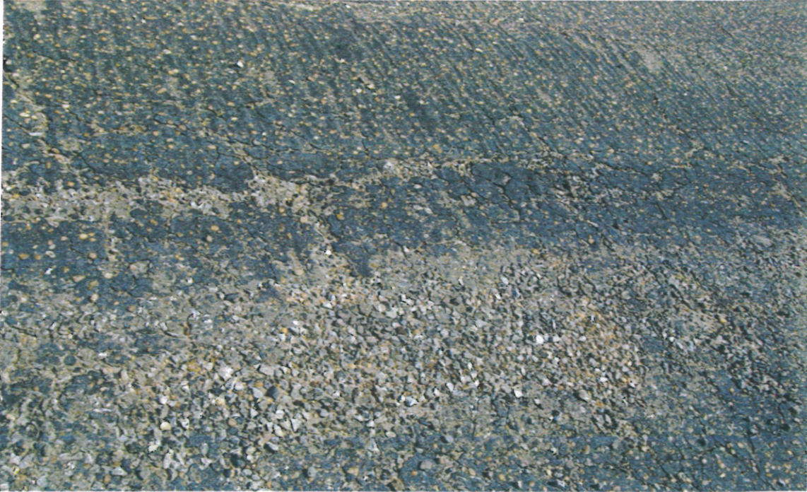
Photo # 6 – Alligator Cracks
