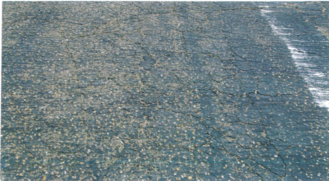
Photo # 6 – Alligator Cracks
