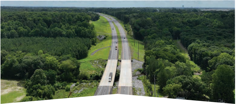
Rebuild Alabama projects added lanes, improved access and strengthened bridges in Fiscal Year 2025.
