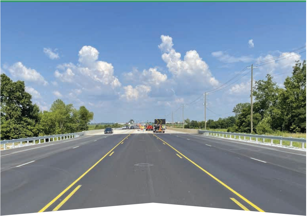
A $13.3 million Rebuild Alabama project reconstructed the two-lane county road as a five-lane state highway between US-31 and I-65.
