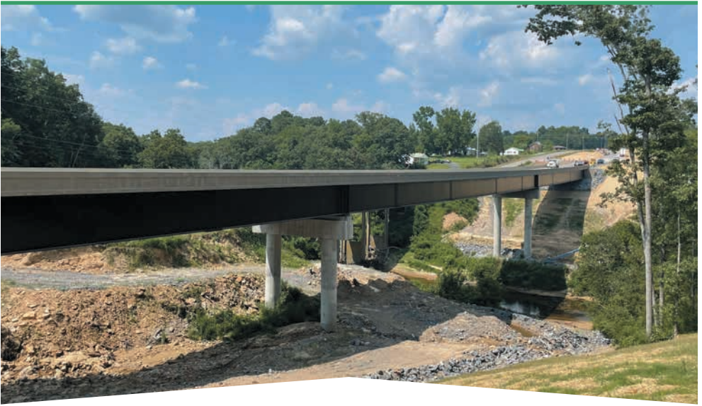
A new bridge on SR-75 over Town Creek in DeKalb County opened in the Summer of 2025.
