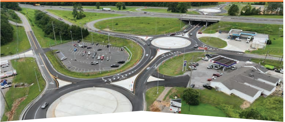
A new series of roundabouts on SR-160 in Blount County designed to reduce serious crashes.
