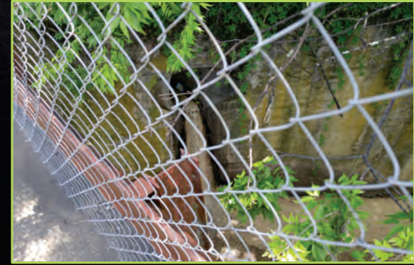
Sanitary Sewer / Grease
