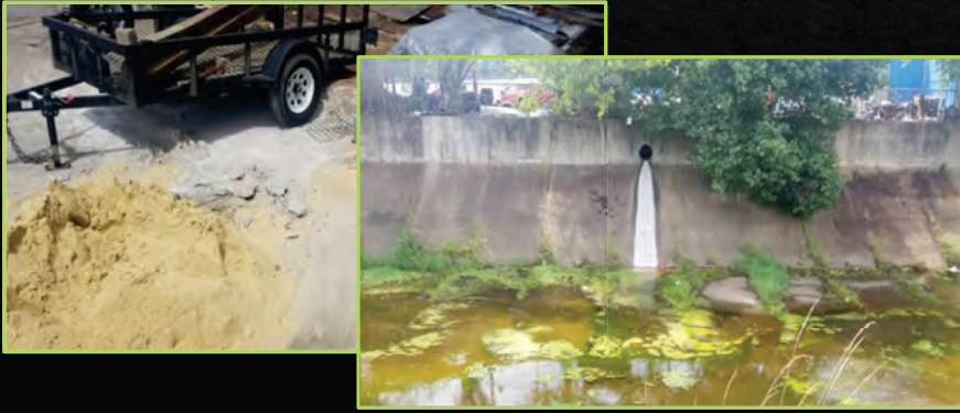
Construction Yard Runoff
