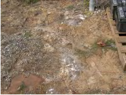
This picture showing battery acid underneath the pallets. Damaged batteries should be placed in containment to prevent the acid from escaping.
