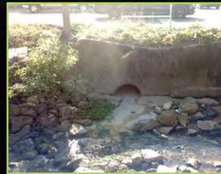
Horizontal Directional Drilling Slurry Runoff
