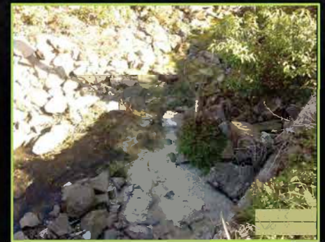
Horizontal Directional Drilling Slurry Runoff
