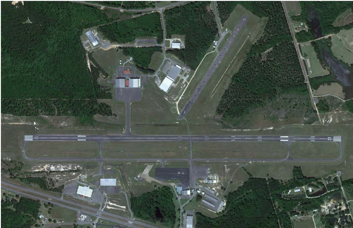
Figure 2.1: South Alabama Regional Airport.
