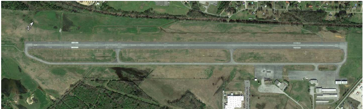
Figure 2.1: Anniston Regional Airport.
