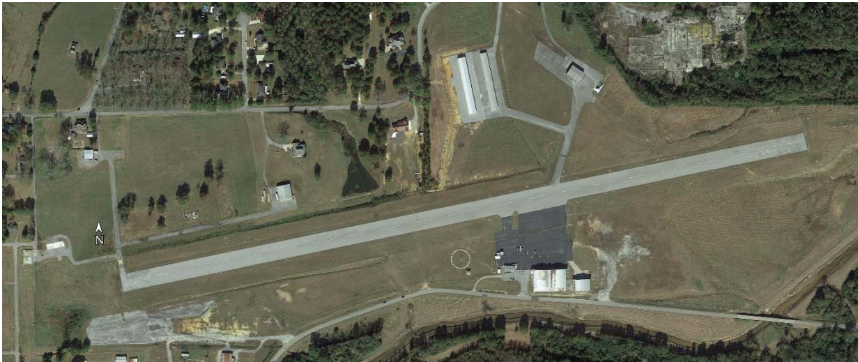
Figure 2.1: Chilton County Airport.
