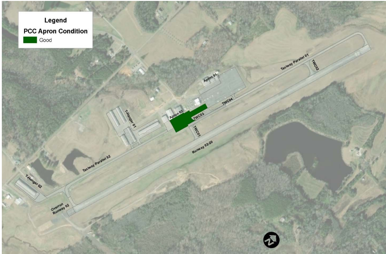
Figure 3.4: PCC Apron Condition Rating.
