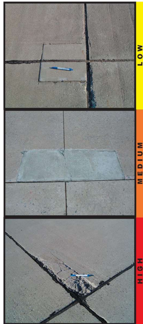
Figure C.14: PCC Small Patch.
