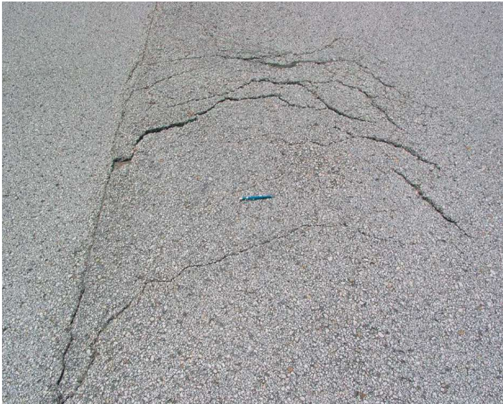
Figure C.10 Slippage Cracking
