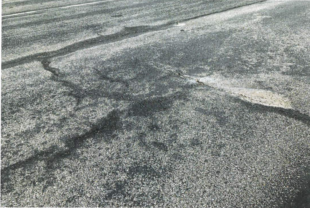
Photo #8 – Taxi-lane Cracking
