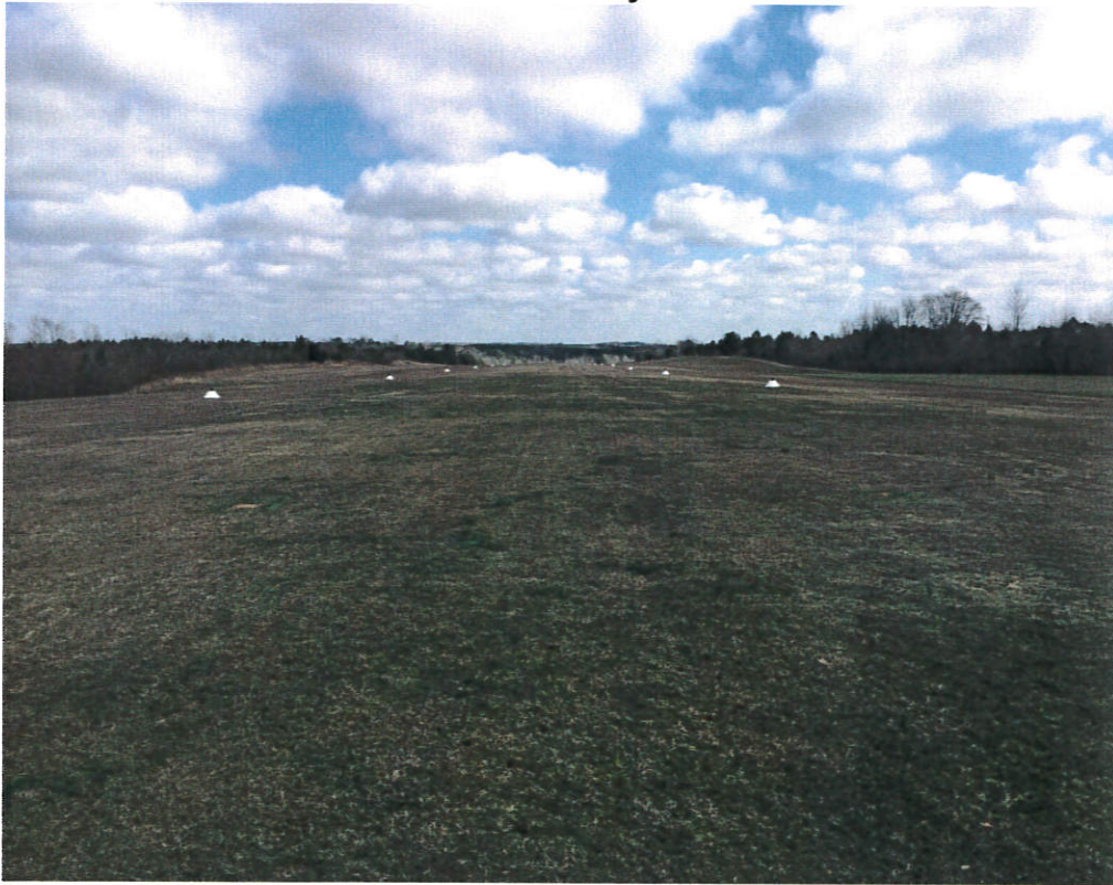
Photo #5- Runway Surface
