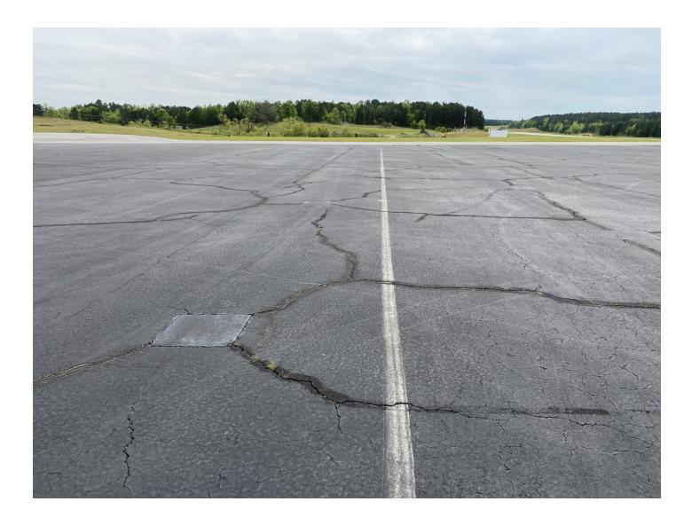
Apron surface is overall in **FAIR** to **POOR** conditions in certain areas. There is extensive longitudinal and transverse cracking. There is alligator cracking in certain areas.
