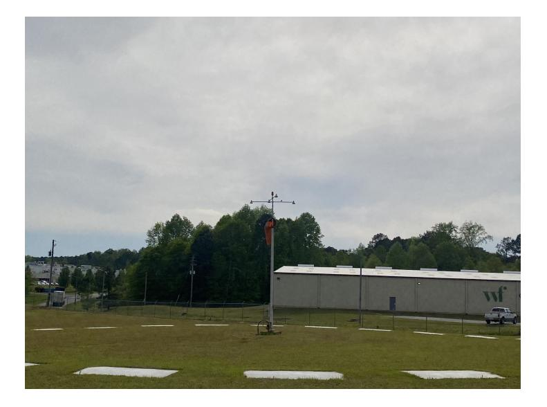
Wind direction indicator is in <u>FAIR</u> condition. Windsock is starting to fade and should be replaced soon.
