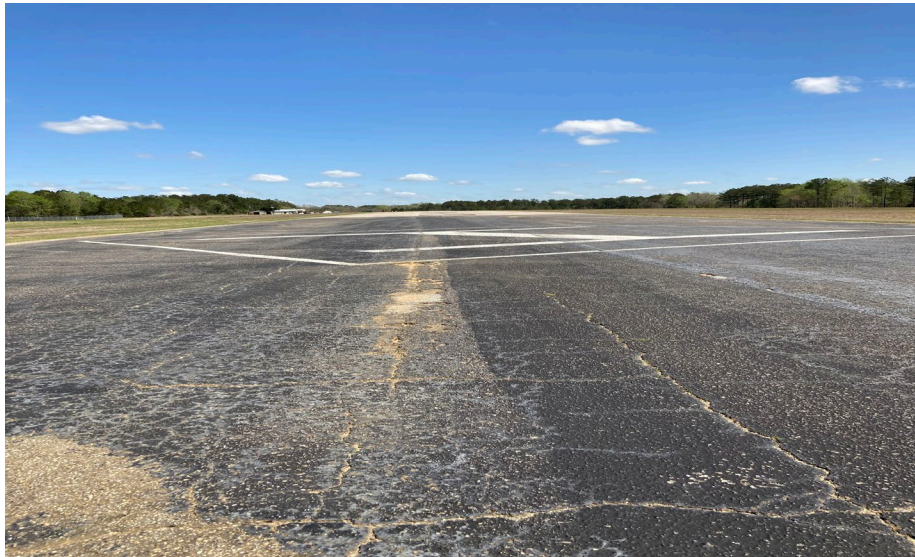
Photo #7-Pavement Failure Around Southern H
