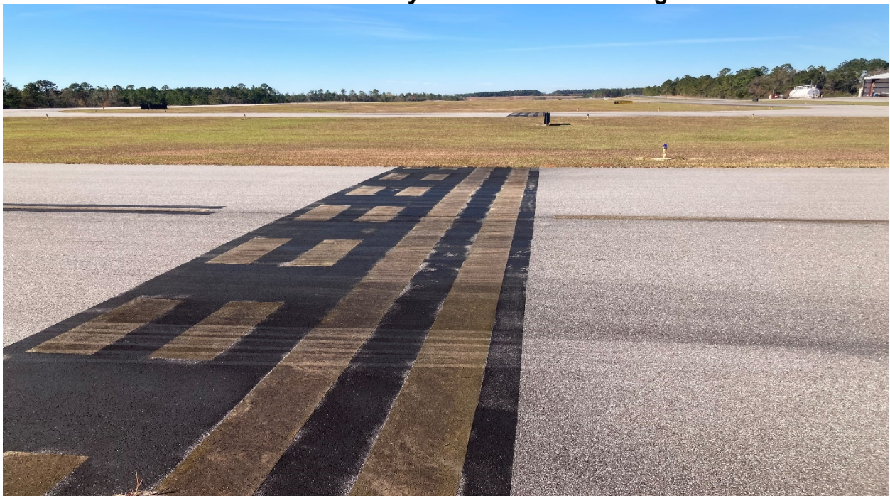
Photo #6 – Runway 26 Hold Short Markings
