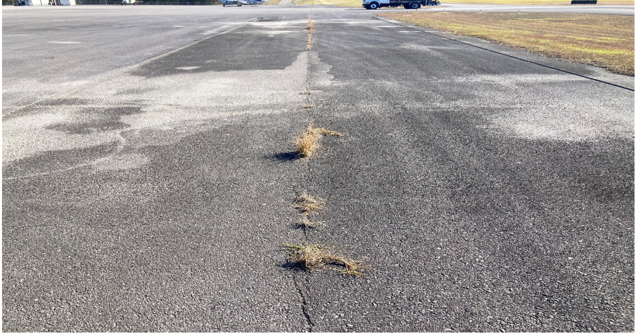
Photo #10 – Main Apron Vegetation
