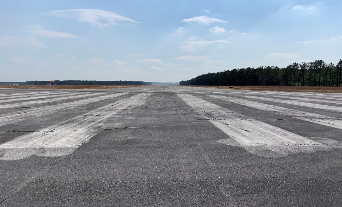
Photo #8 – Runway 12 Markings
