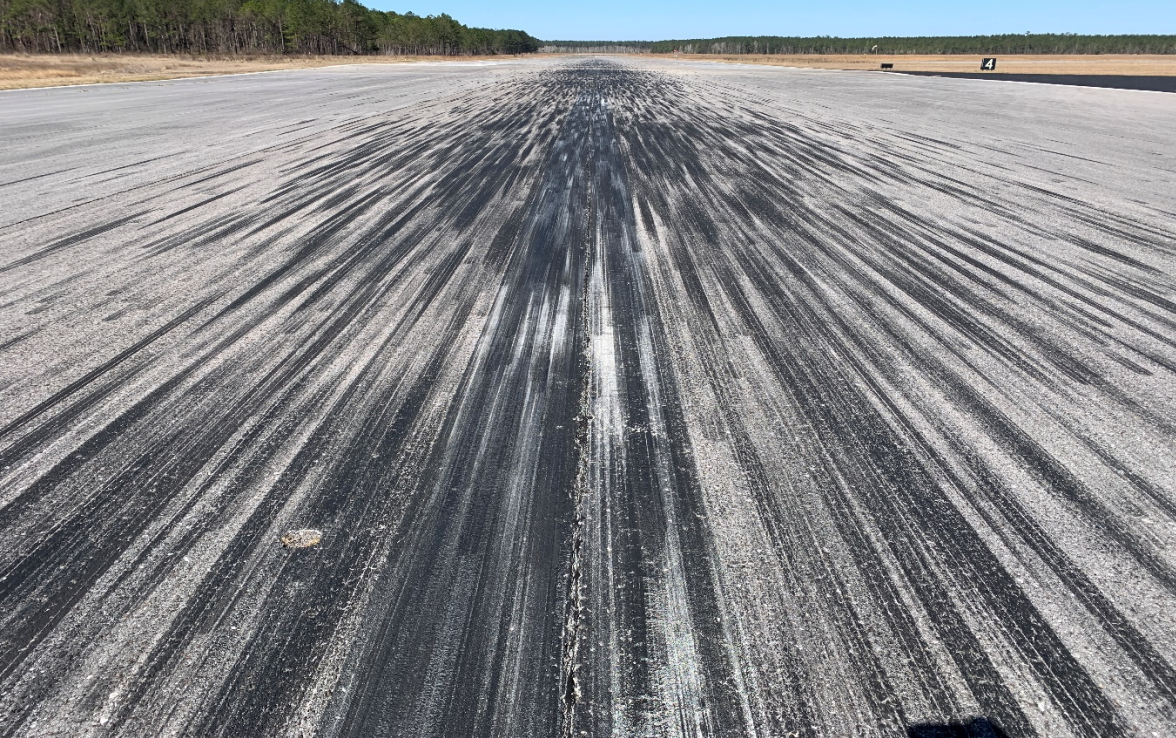
Photo #9—Runway 12/30 Centerline Stripes
