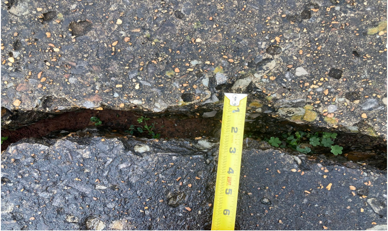
Photo #27 – Runway 18/36 Cracking
