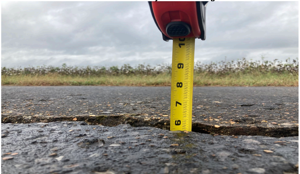
Photo #27 – Runway 18/36 Cracking
