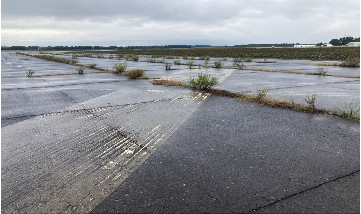
Photo #12 – Faded X's on Closed Runway
