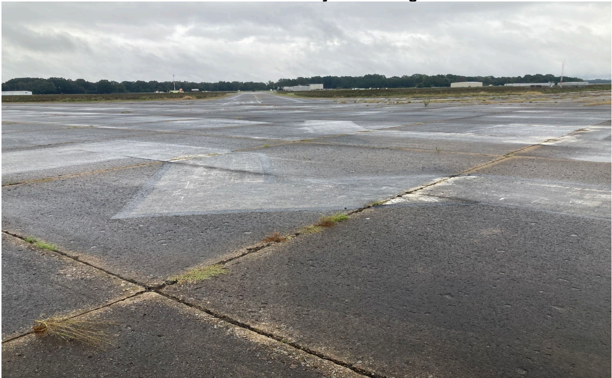
Photo #9 – Runway 36 Markings
