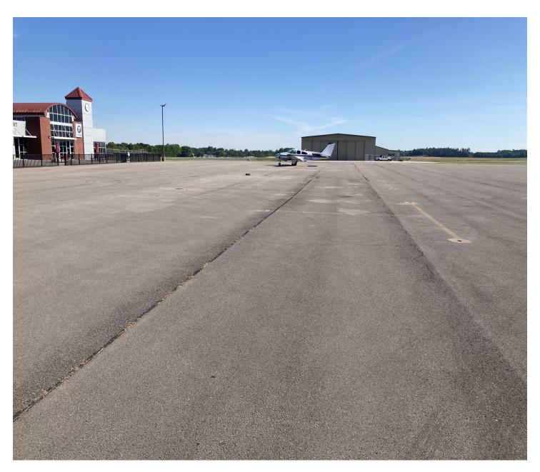
The Terminal Apron is in <u>FAIR</u> condition due to minor cracking and vegetation growth.
