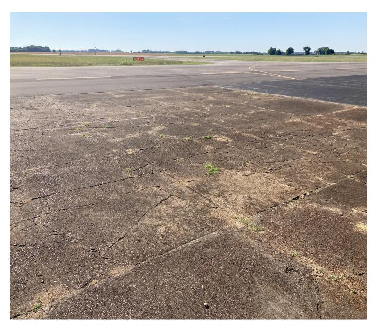
The old North Alabama Aviation Apron is in **POOR** condition due to widespread cracking and vegetation growth.
