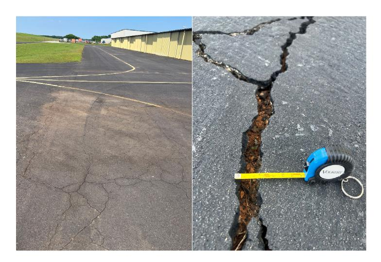
The taxilane surface near the hangars is in **POOR** condition and is experiencing extensive longitudinal, transverse, and alligator cracking in certain areas.
