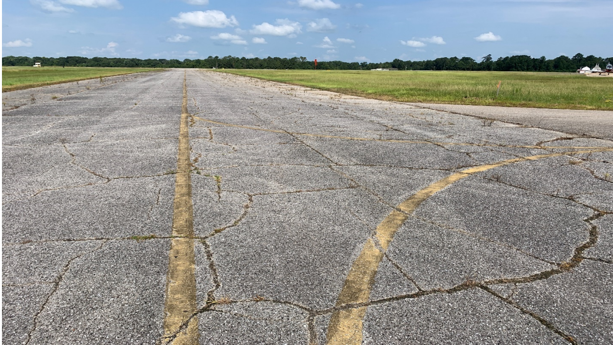
Photo #6—Taxiway Markings
