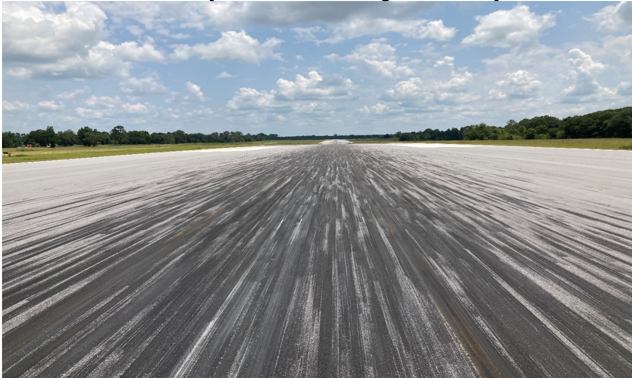
Photo #5 – Runway 10 Centerline Markings Obscured by Rubber
