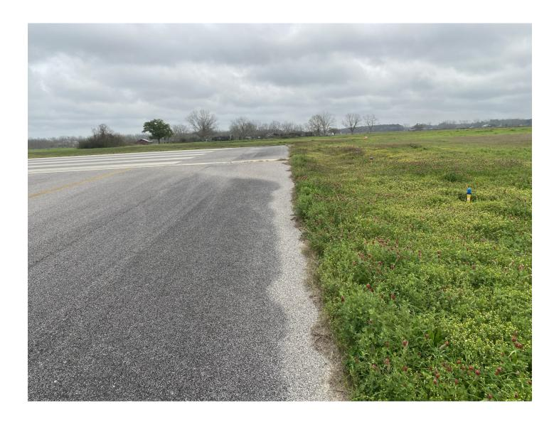
Maintenance Required: Remove grass growing over the pavement edges. Edge of pavement should be visible. Grass encroaching on pavement edges can potentially cause standing water leading to damage and deterioration of the pavement.
