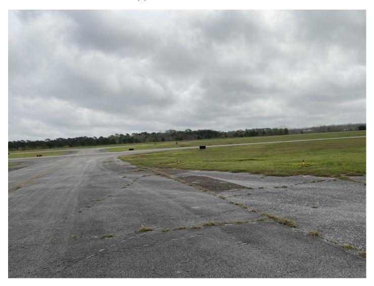
Taxiway surface is generally in <u>FAIR</u> condition. There are portions of some taxiways in <u>POOR</u> condition. Taxiway surface in poor condition is experiencing moderate cracking and vegetation growth.
