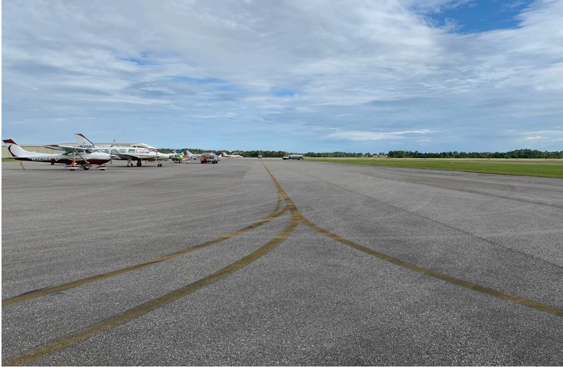
Photo #11 – Main Parking Apron
