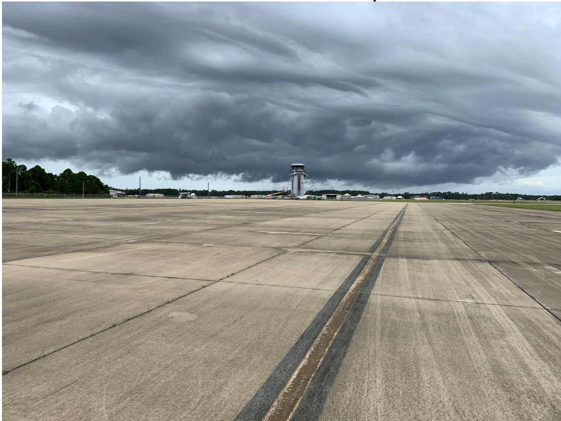
Photo #10 – New Concrete Apron
