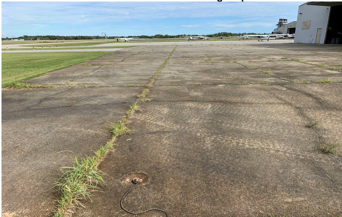
Photo# 12 – Maintenance Hangar Apron
