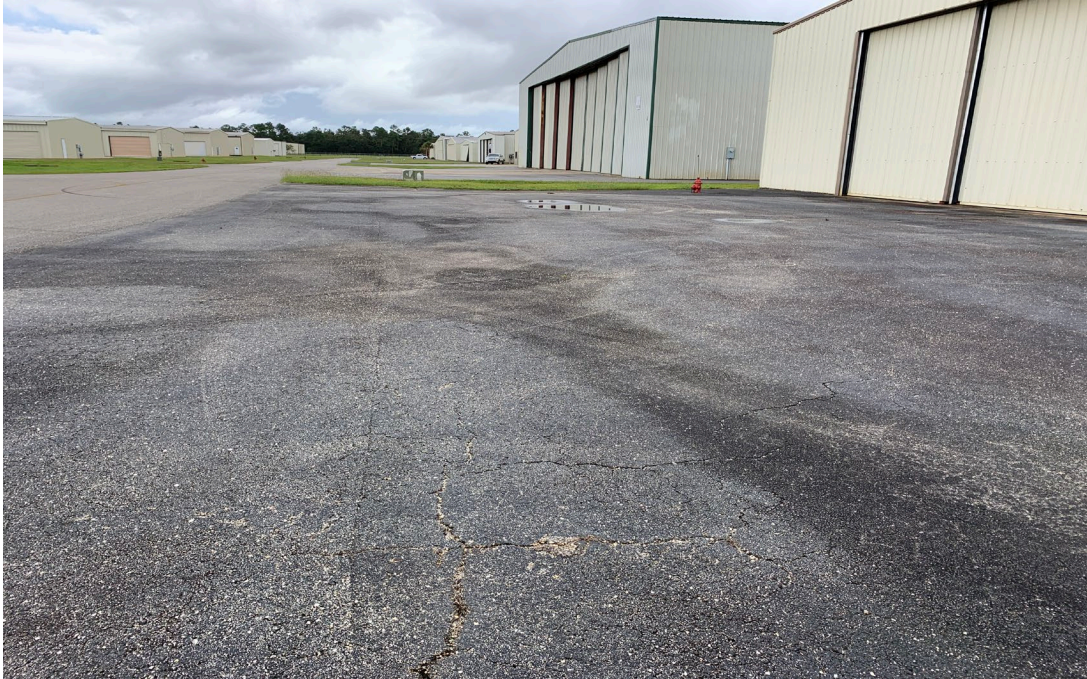
Photo #13 – Hangar Apron (West Side)
