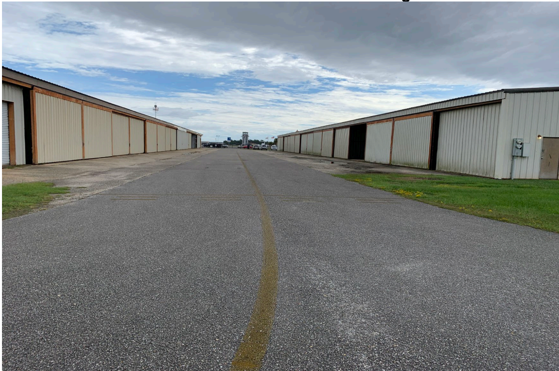
Photo #8 – West Taxi Lane Markings
