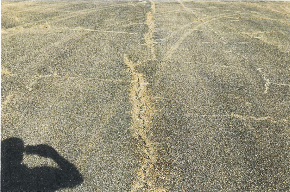
Photo #11 – Secondary (Old) Ramp Raveling
