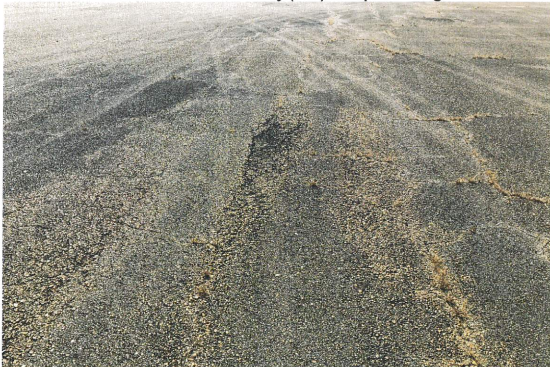
Photo #11 – Secondary (Old) Ramp Raveling
