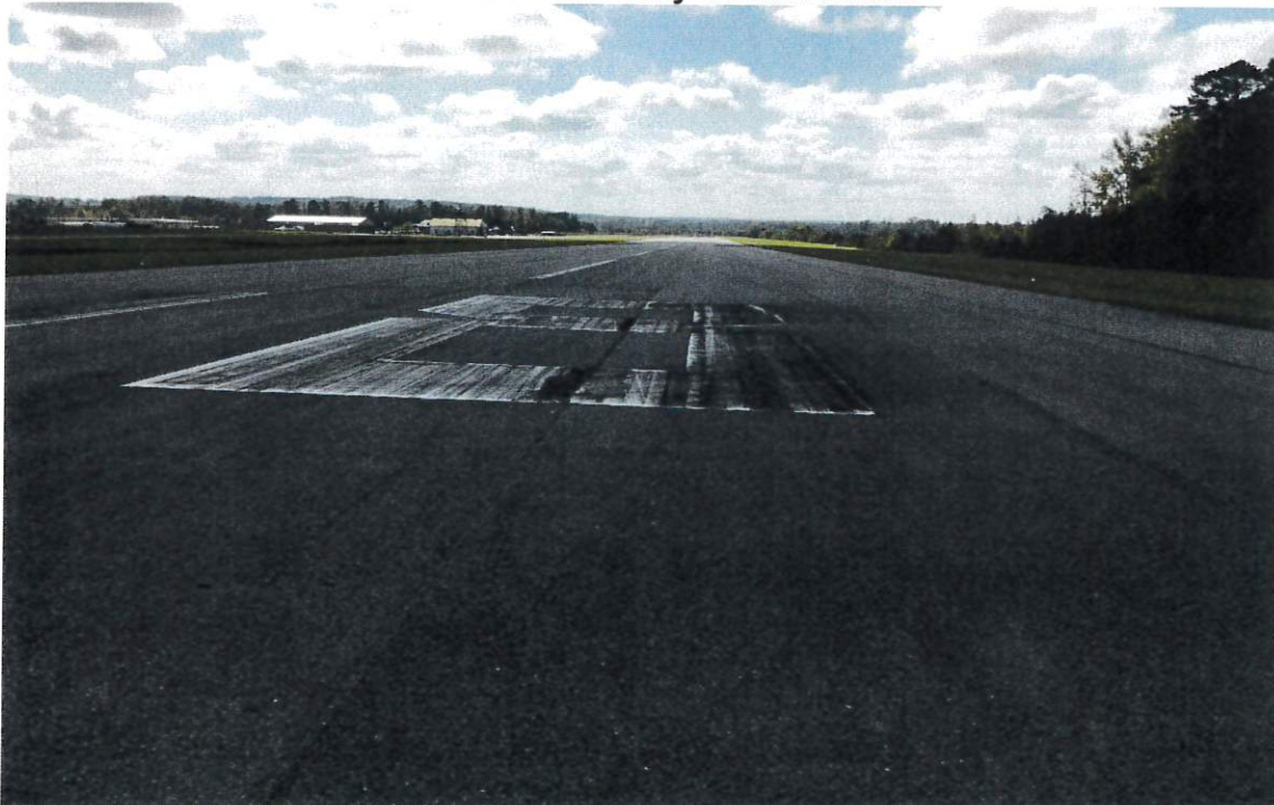
Photo #5—Runway 18 Identifiers
