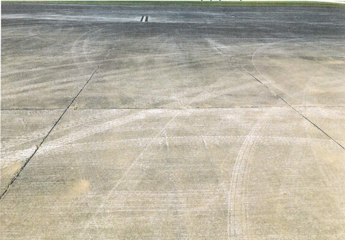
Photo #9 – Main Ramp (Apron)
